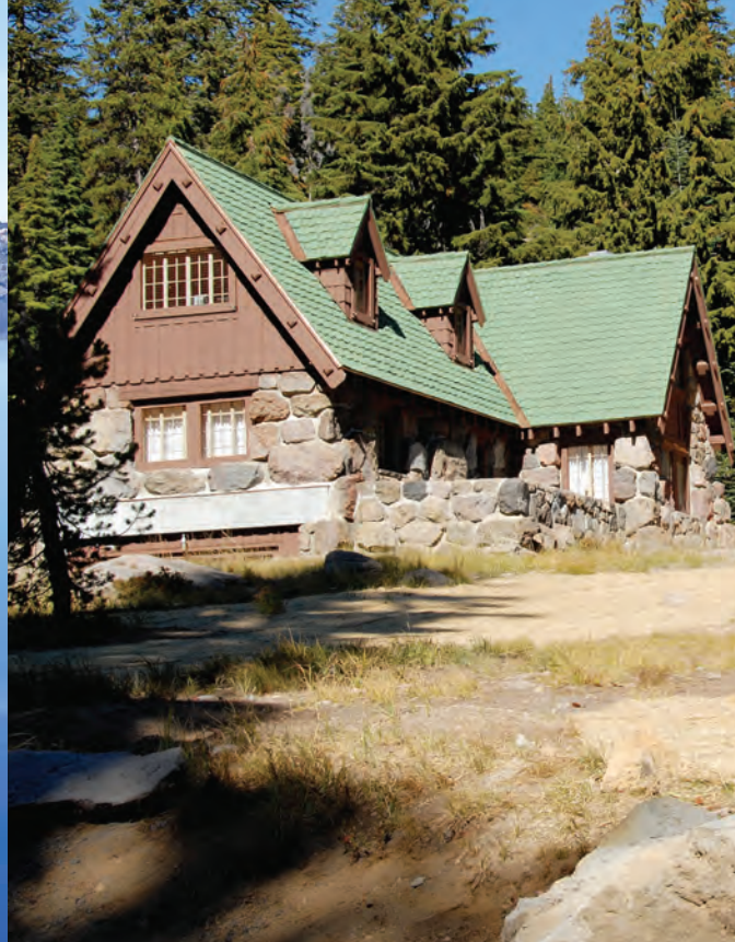
The Science and Learning Center is housed in the Superintendent's
